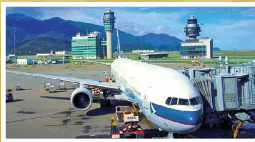
Chek Lap Kok Airport opened for commercial operations in 1998. Its 12.48 km 2 platform was formed by levelling neighbouring Lam Chau Island and land reclamation on the original Chep Lap Kok Island.
